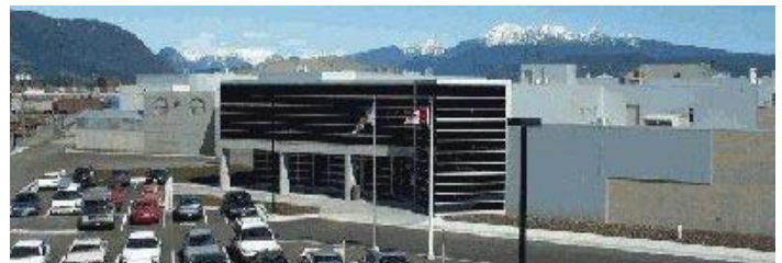
North Fraser Pre-Trial Centre (NFPC).
